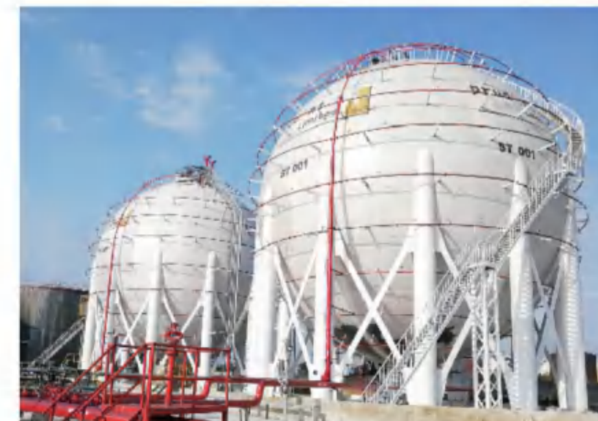
Nigeria 2x6000m 3 Spherical Tank
